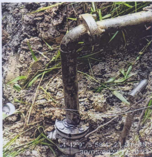
SPILL POINT ( Before excavation )
